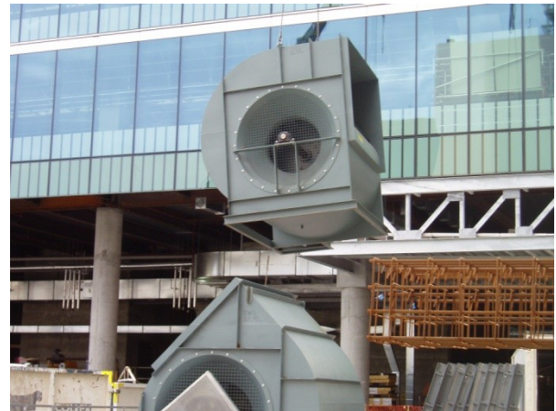
Figure 2. AHU 18-1 SA fans being lifted into position during construction
